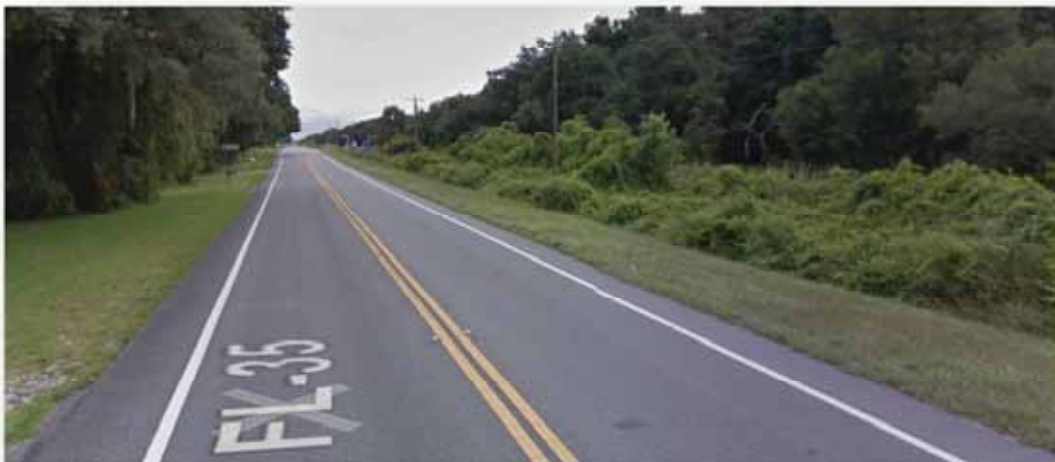
Figure 6.5: Existing Paved Shoulders along US 301 (SR 35)
