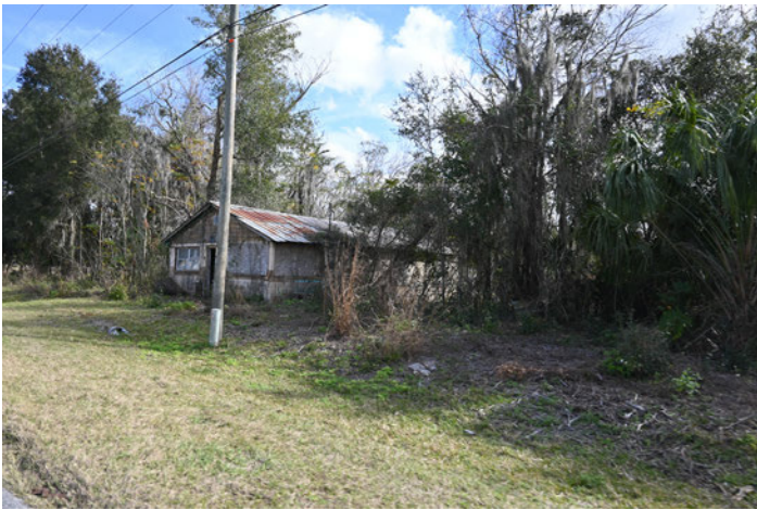
8SM01343_o Facing Southeast
