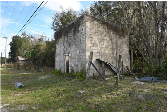
8SM01343_m Facing Southeast
