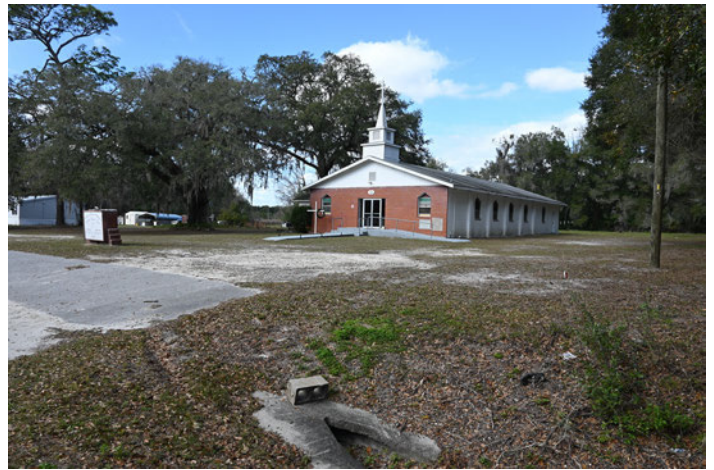
8SM01343_j Facing Southwest
