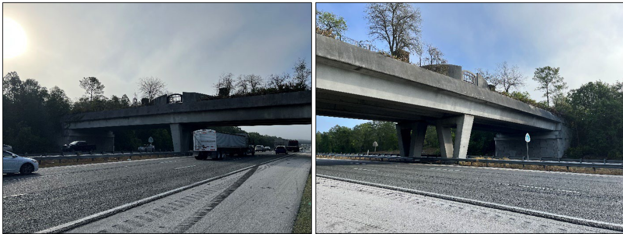
Figure 52. Representative views of 8MR03410. Left: facing southeast. Right: facing southwest.
