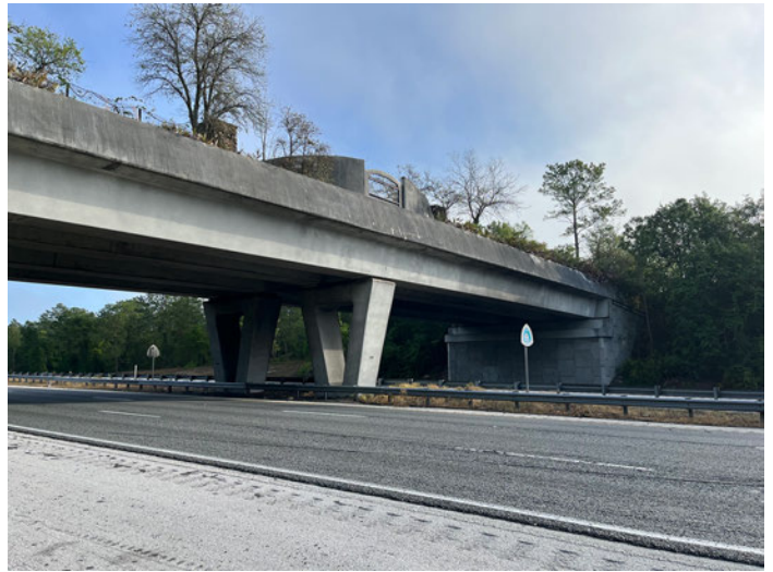
8MR03410_d Facing Southwest
