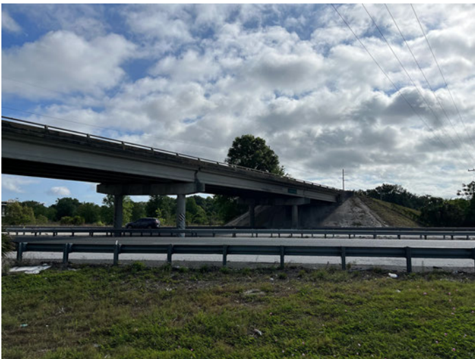
8SM01393_c Facing Northeast
