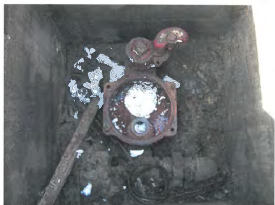
View of a UST filled with foam (permafill)
