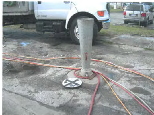
View of degassing a UST before closure in place
