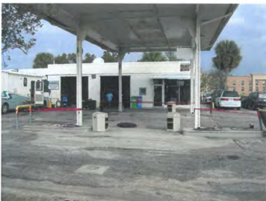
View of removed dispensers from fuel islands
