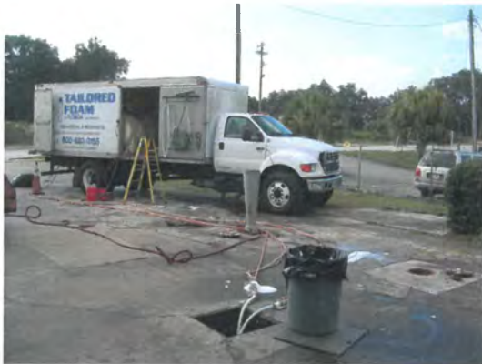
View of UST closure in place
