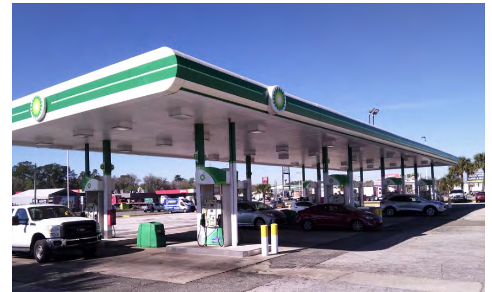
View of the fueling canopy and gas pumps on-site.
