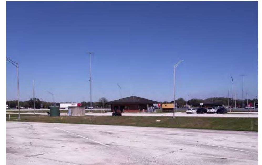
Looking east towards the emergency generator (yellow) and belly tank (black).
