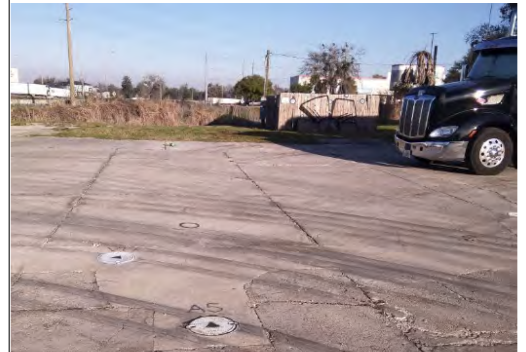
Looking north at the area of the former gas station. The remediation system trailer is behind the fence in the background.
