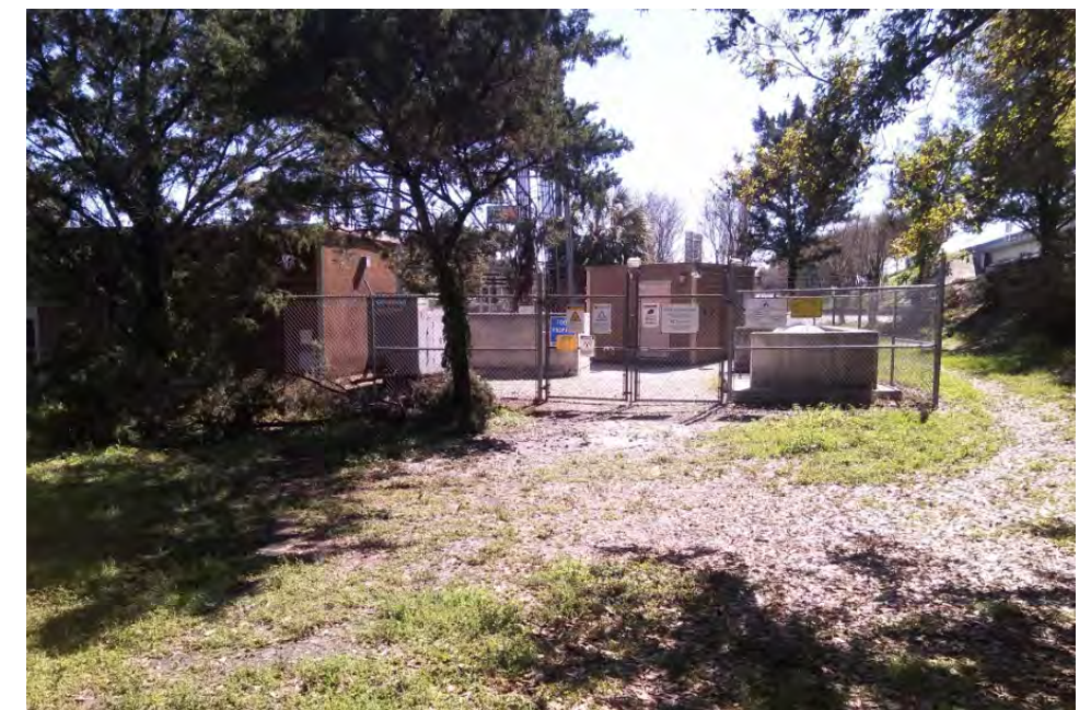
View of the radio tower base on-site.
