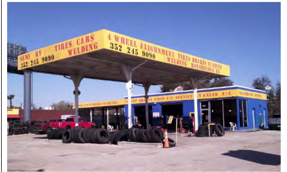
Looking north at the former gas station fueling canopy.
