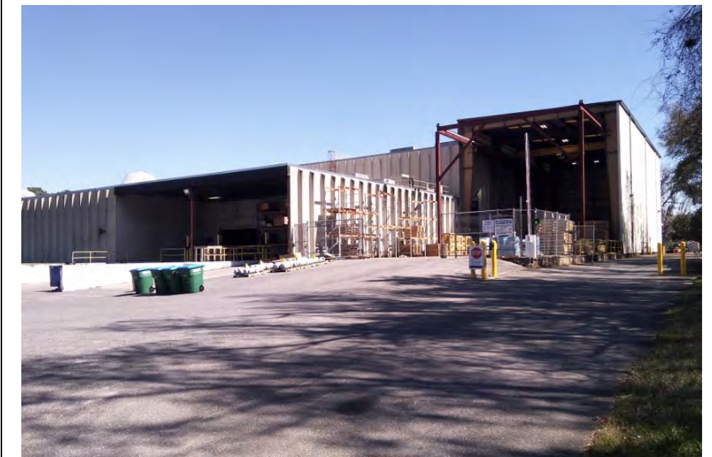
View of the warehouse building on-site.
