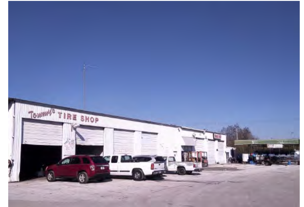
Looking north at the auto repair shop.
