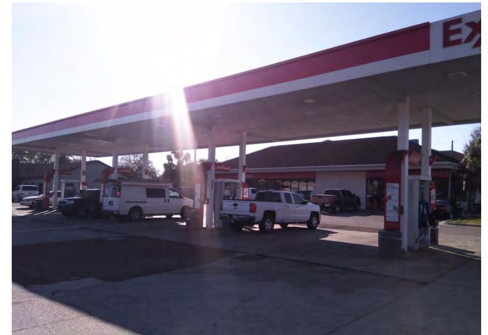
View of the gas station and fueling canopy.
