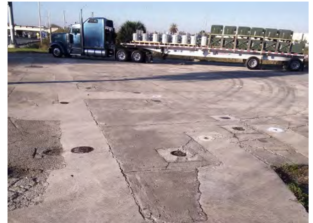
View of an area of monitoring wells.
