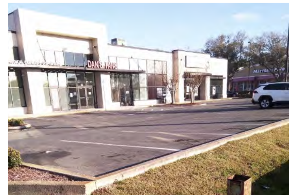
Looking north at the area of the former gas station.
