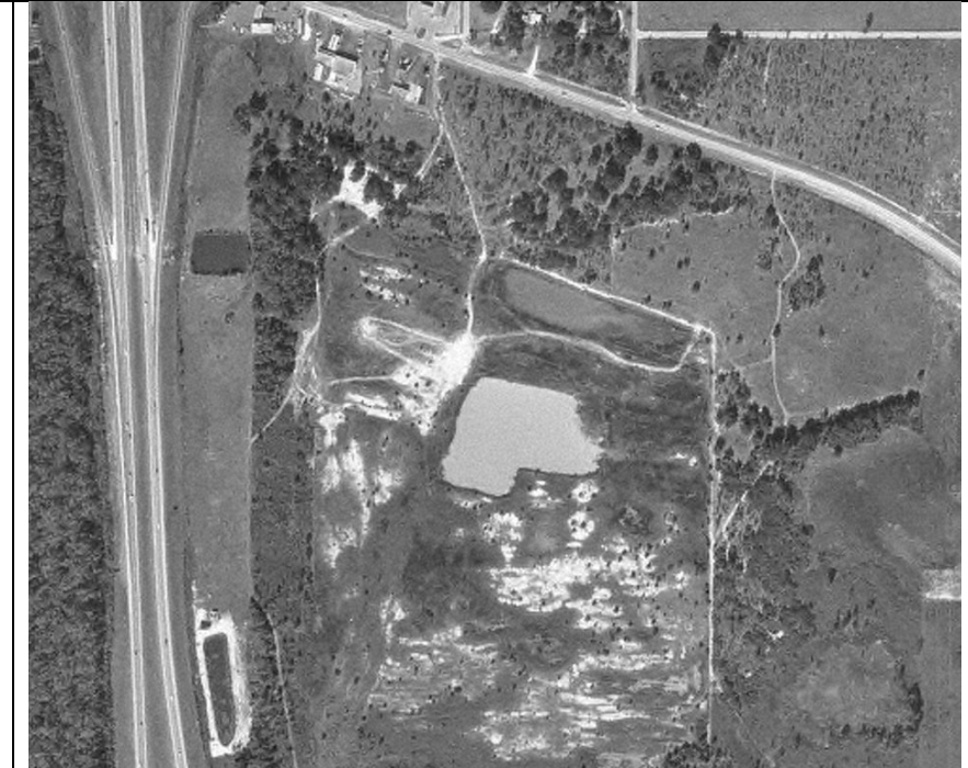
View of an area of excavation located southeast of the I-75 and SR 44 interchange, on the 1973 aerial photograph.
