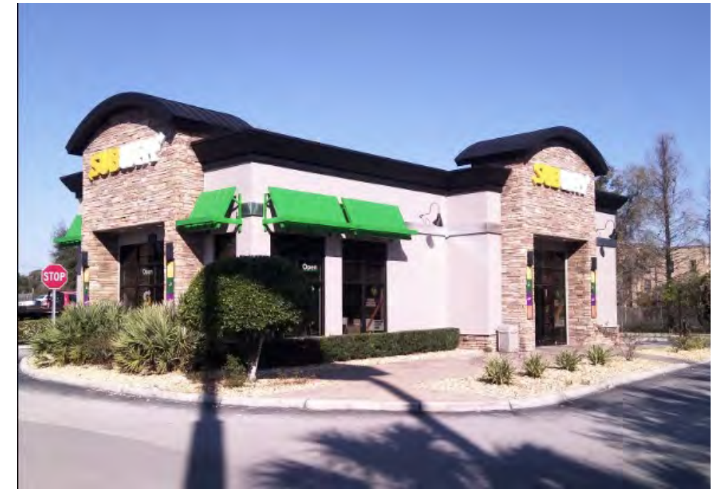
Looking northwest at the current restaurant building.
