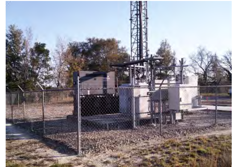
View of the base of the radio tower.
