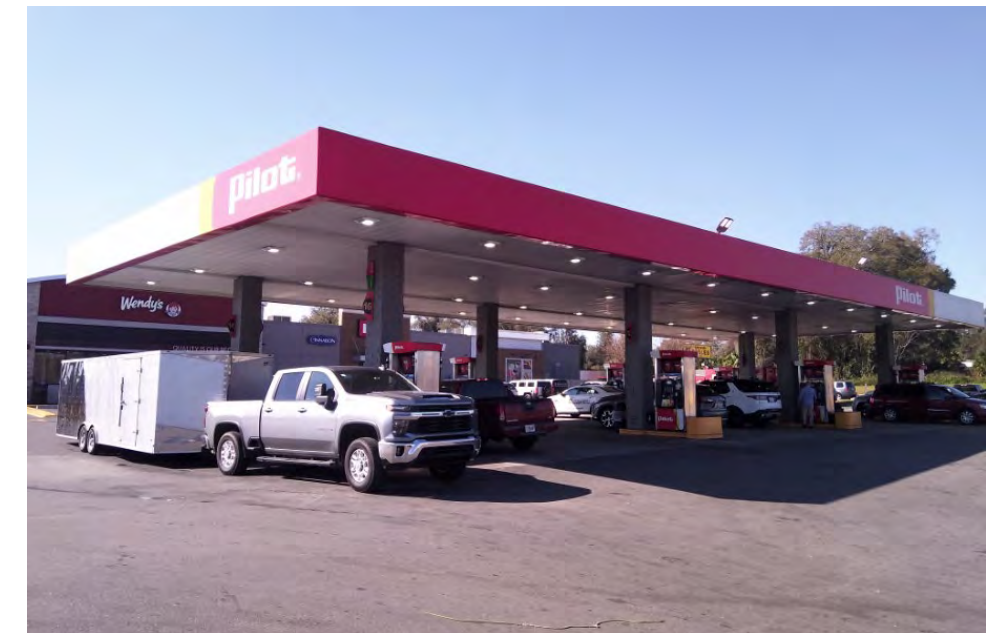
View of the fueling canopy and gas pumps.
