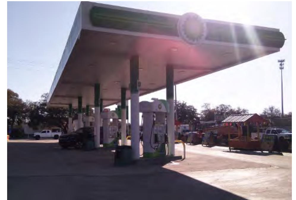
View of the fueling canopy and gas pumps on-site.
