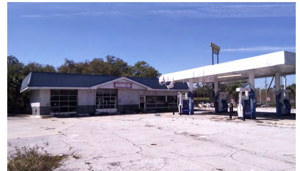
Looking south at the former gas station and fueling pumps. A monitoring well is in the foreground.
