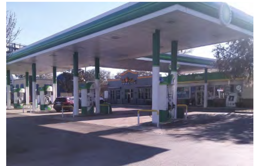
View of the gas station and fueling canopy on-site.
