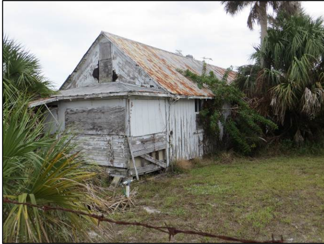
Figure 25. Example of Shotgun style: Resource 8BR03090, facing southeast.
