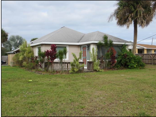
Figure 22. Example of Minimal Traditional style: Resource 8BR03096, facing northeast.
