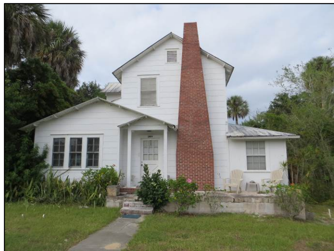
Figure 26. Example of Tudor Revival style: Resource 8BR03079, facing north.
