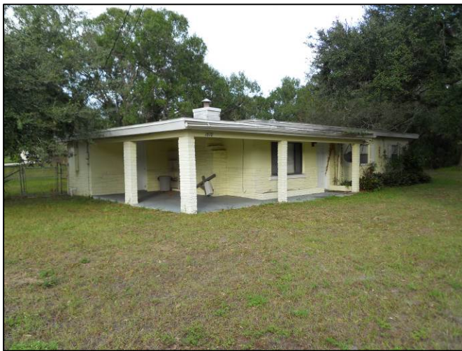
Figure 21. Example of Ranch style: Resource 8BR03114, facing northeast.
