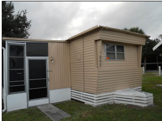
Figure 23. Example of a mobile home: Resource 8BR03121, facing west.
