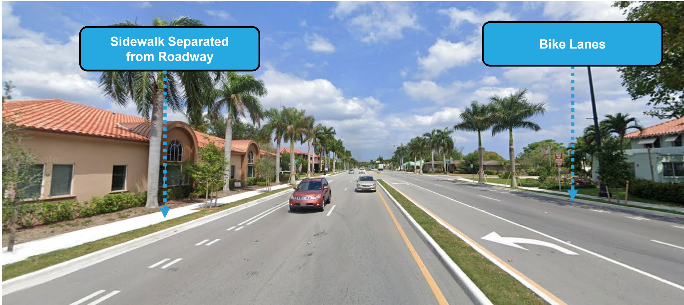
Enhanced Condition of SR 810 in Deerfield Beach, Florida
