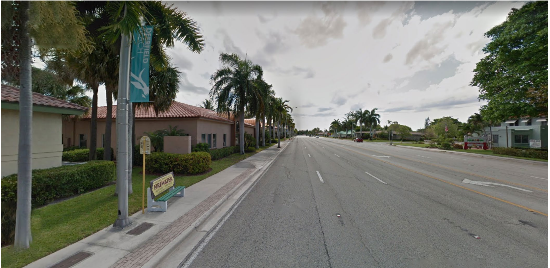
Initial Condition of SR 810 in Deerfield Beach, Florida
