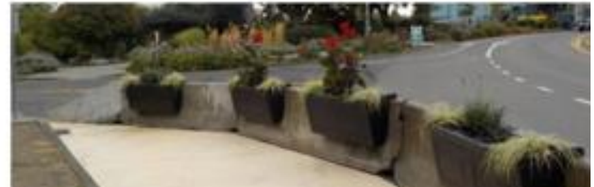
Concrete Barrier Wall with Sidewalk
