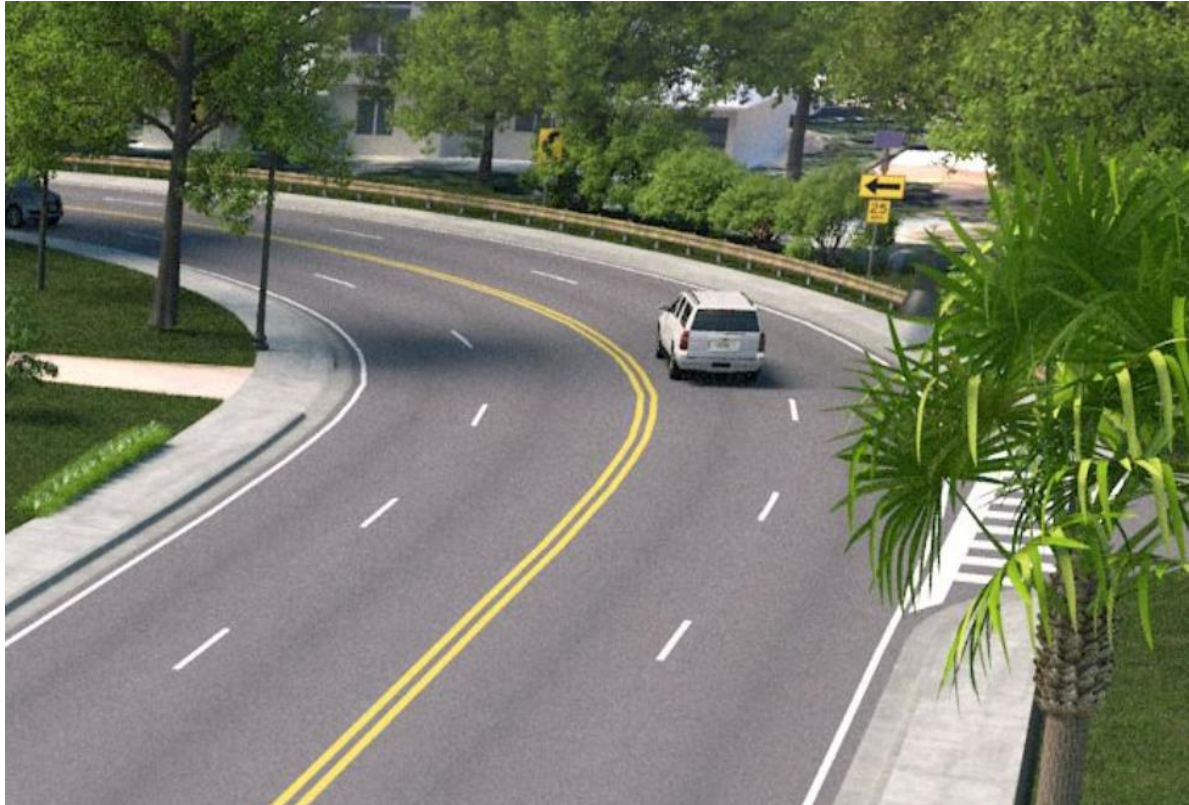
Westbound approaching Brewers Curve EXISTING
