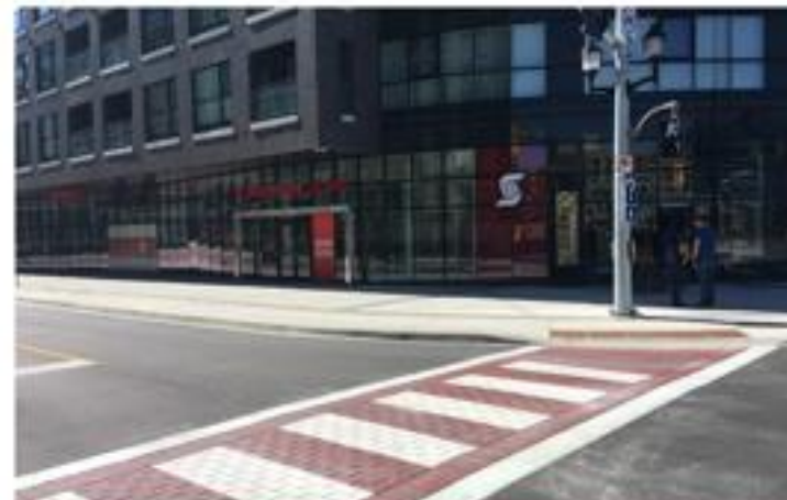
High Visibility Crosswalks
