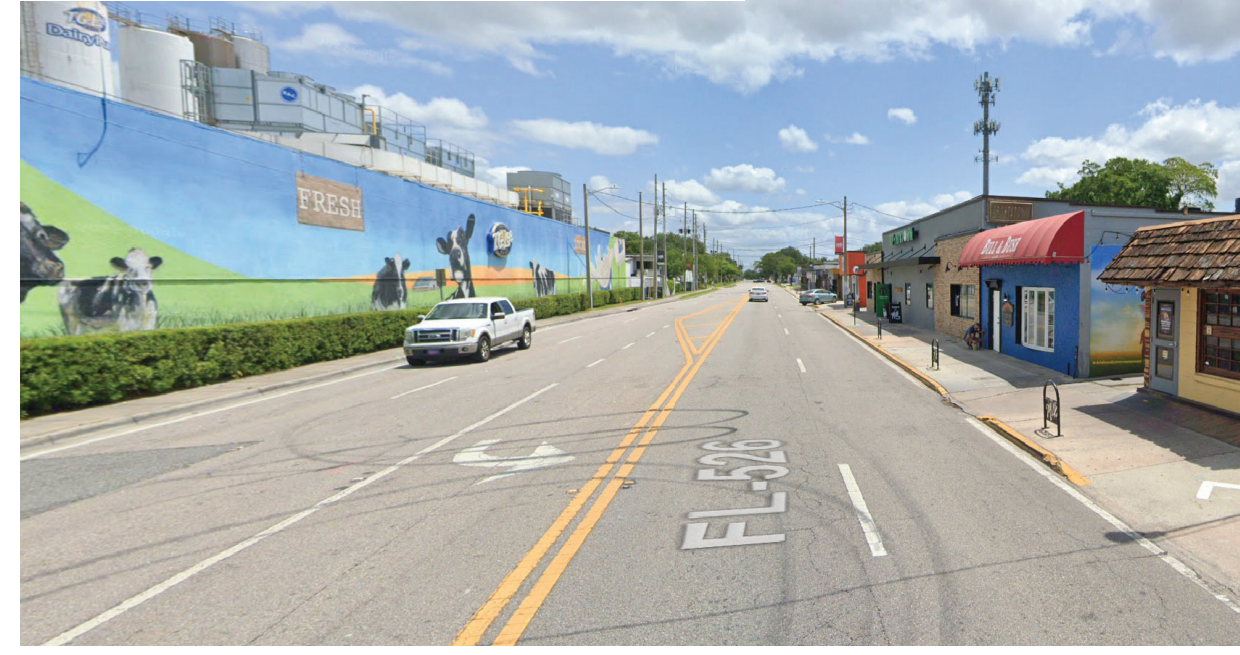
Existing Conditions Looking East
