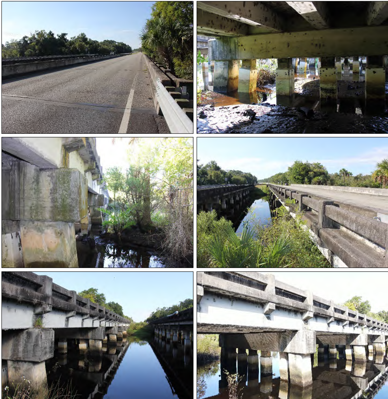
Figure 3. Representative views of Resource 8FL01008/8SJ08262. Deck and roadway, facing southeast (top left); underside with girders and piers, facing southeast (top right); west side of structure, facing south (middle left); railing along east side, facing south (middle right); railing and east side, facing north (bottom left); east side and piers, facing northwest (bottom right).
