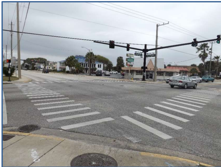
Looking west at US 92/SR 600/ISB from the SR 441/Peninsula Dr intersection.
