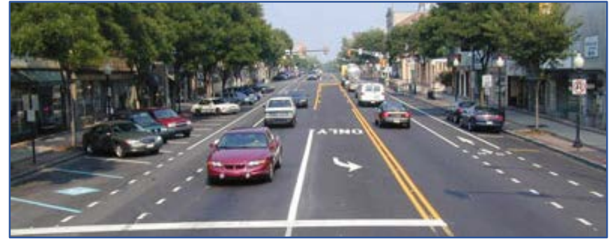
An example of bike lanes in conjunction with on-street parking (Pottstown, PA)
