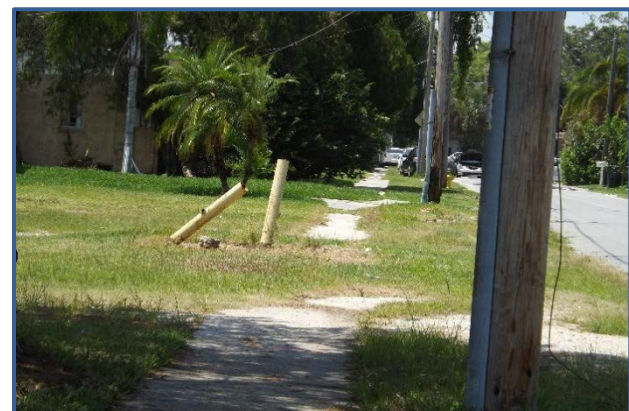
Sidewalk gaps exist on the west side of Jefferson St.
