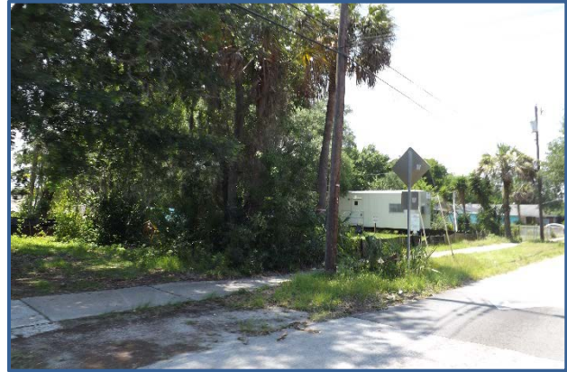
Vegetation obstructs the sidewalk on Keech St.
