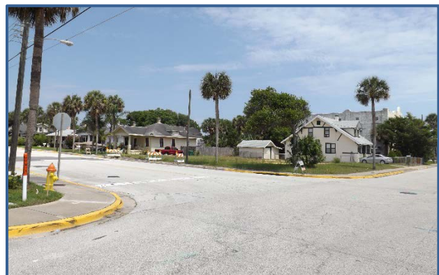
There are no ADA accessible sidewalk ramps at the intersection of Grandview Ave and Goodall Ave.
