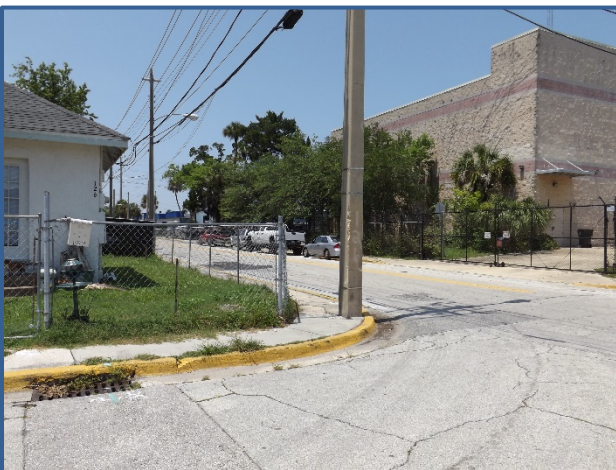
There are no ADA accessible sidewalk ramps at the intersection of Charles St and West St.
