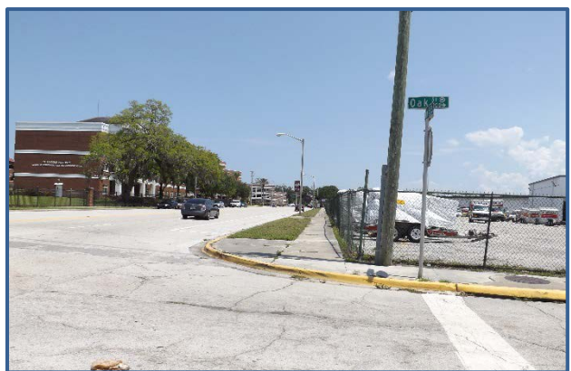
There are no ADA accessible ramps at the intersection of Dr. MLK Blvd and Eldorado St.
