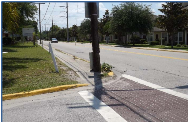
A utility pole obstructs the sidewalk on Dr. Mary McLeod Bethune Blvd.
