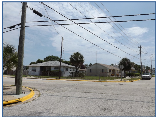
Three of four corners at the intersection of Grandview Ave and Lenox Ave lack ADA accessible sidewalk ramps.
