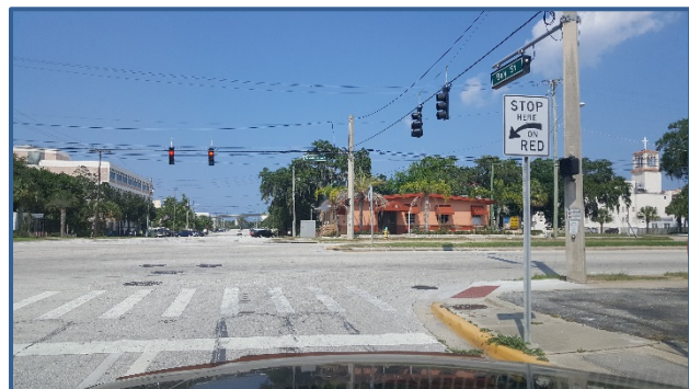
The intersection of US 1/Ridgewood Ave and Bay St lacks a crosswalk on the south side.
