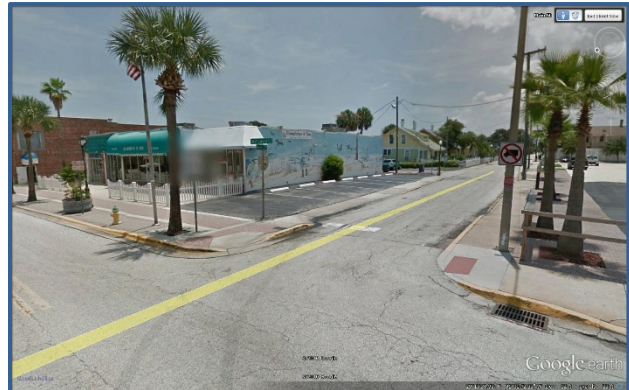
The intersection of Main St and Hollywood Ave does not have a marked crosswalk.
