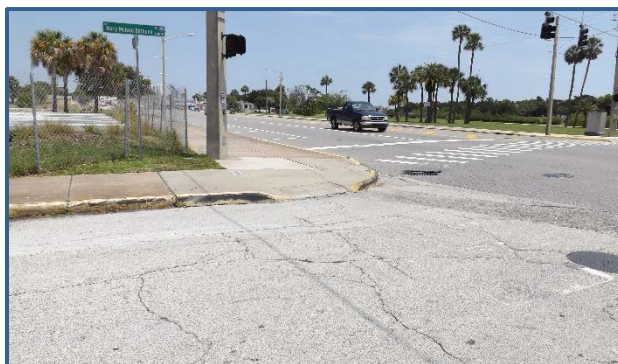
A faded marked crosswalk at Beach St and Dr. Mary McLeod Bethune Blvd.
