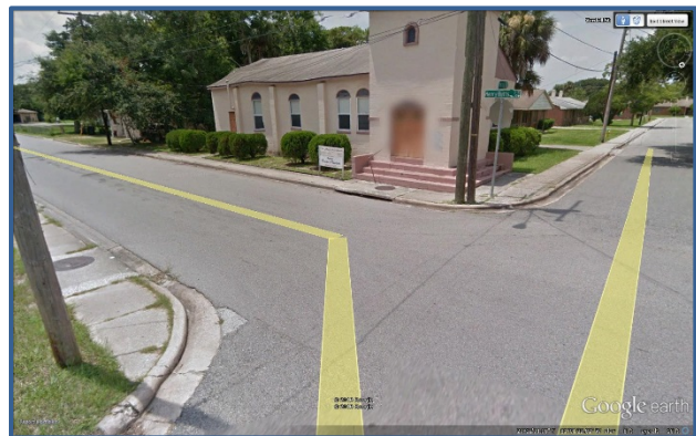
There are no ADA accessible sidewalk ramps at Henry Butts Dr and Verdell St.
