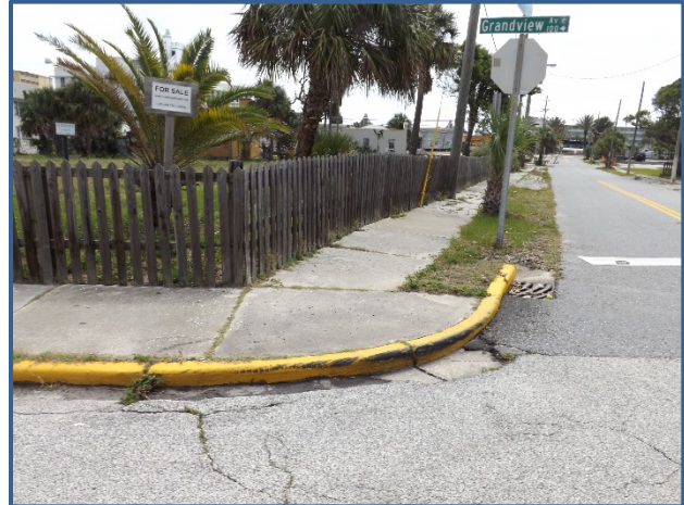
There are no ADA accessible sidewalk ramps at the intersection of Grandview Ave and 5 th Ave.
