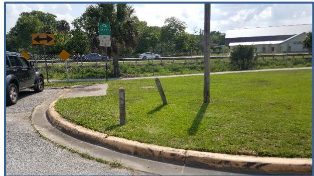
There is a gap in the sidewalk network between the SR 5A/Nova Rd multi-use path and Jean St.
