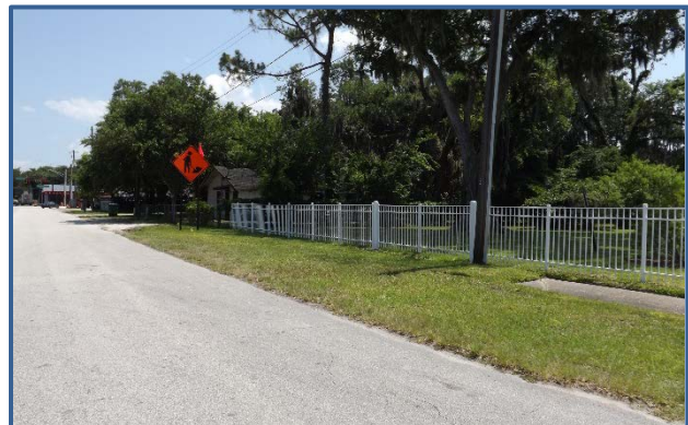
A sidewalk on Adams St abruptly ends.
