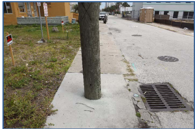
A utility pole obstructs the sidewalk on Coates Street.
