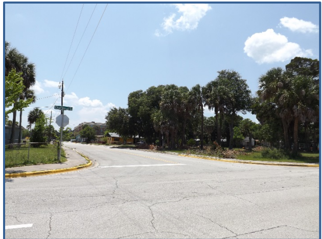
Several intersections along the McLeod Ave corridor lack ADA accessible sidewalk ramps.
