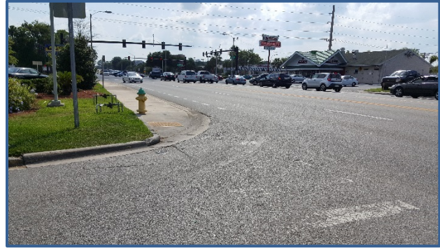
An example of a faded marked crosswalk at US 92/SR 600/ISB and Jean St.
