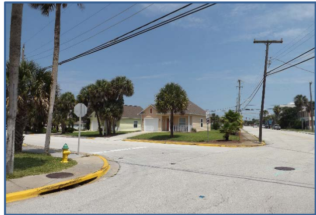
There are no ADA accessible sidewalk ramps on the west side of the intersection of Grandview Ave and Vermont Ave.
