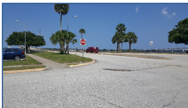
There is no marked crosswalk at Fairview Ave and Bowman Ave.
