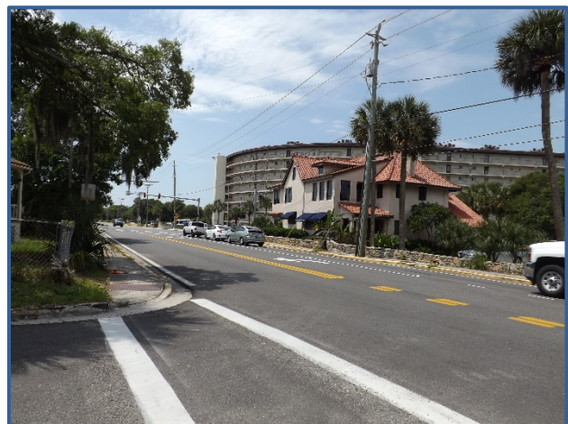
There are no bicycle facilities on SR 441/Peninsula Dr between Phoenix Ave and Silver Beach Ave.
