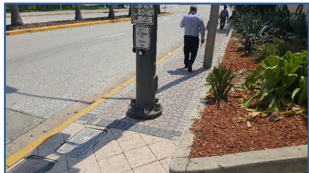
A traffic signal impacts the sidewalk width on Earl St.
