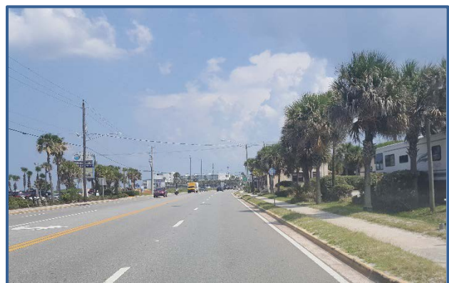
SR A1A/Atlantic Ave does not have marked pedestrian crossings between Revilo Blvd and Silver Beach Ave.
