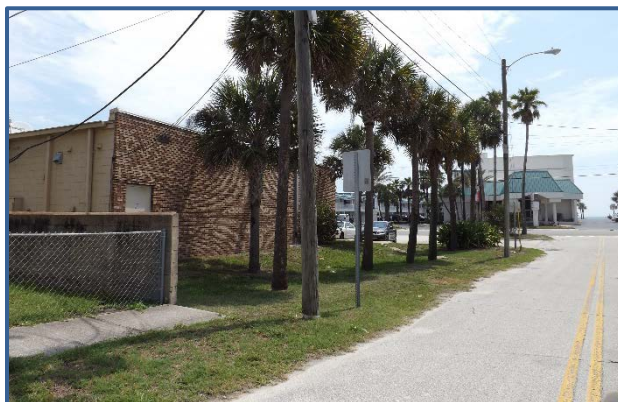
A gap in the sidewalk network on Phoenix Ave.
