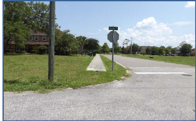
This sidewalk abruptly ends at Oak St and Fulton St.
