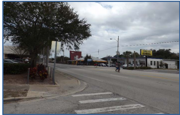
There is a lack of marked pedestrian crossings on US 92/SR 600/ISB in this section.
