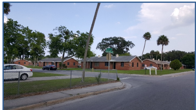
There is no ADA accessible sidewalk ramp at the northeast corner of Lockhart St and Hawk St.
