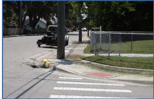
A utility pole obstructs the sidewalk on Marion St.
