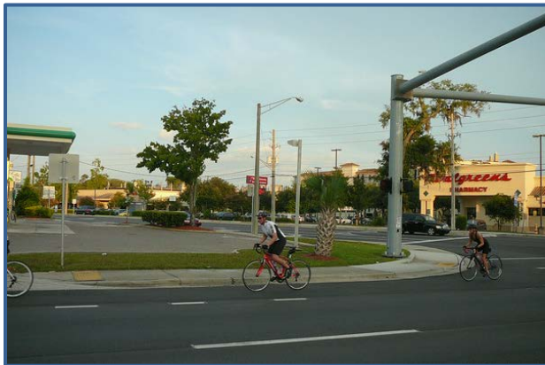
A view of SR 13/San Jose Blvd, shortly after the completion of a FDOT milling and resurfacing project. As a part of the project, existing roadway lane widths were "right-sized" to create space for new bicycle lanes. Photographs courtesy of Moderncities.com and dated August 2014.
