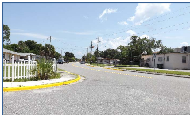
There are no ADA accessible ramps at the intersection of Walnut St and Weaver St.
