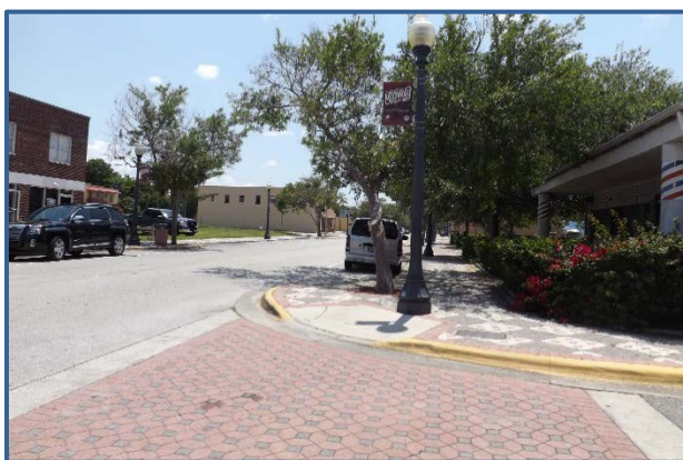
A streetlight obstructs the sidewalk ramp at Weaver St.
