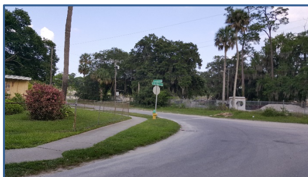
There are no ADA accessible sidewalk ramps at the intersection of Loomis Ave and Lockhart St.
