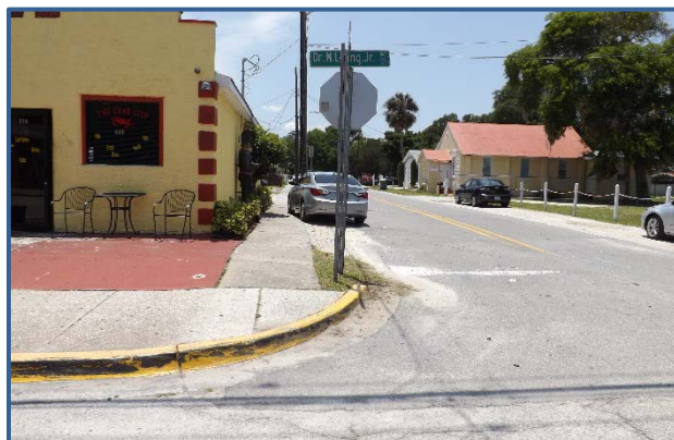
There are no ADA accessible ramps at the intersection of Dr. MLK Blvd and Cherry St.
