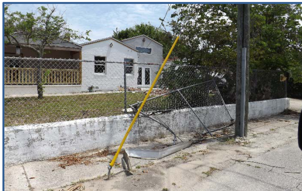
A broken fence obstructs the sidewalk on Goodall Ave.
