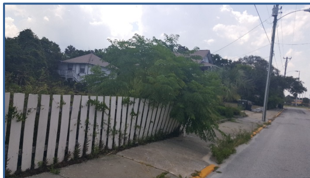
Vegetation obstructs the sidewalk on Hollywood Ave.
