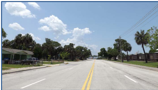
Charles St is a 4-lane thoroughfare with an AADT count of less than 10,000.
