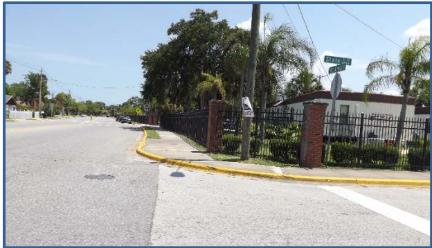
There are no ADA accessible ramps at intersections along State St.
