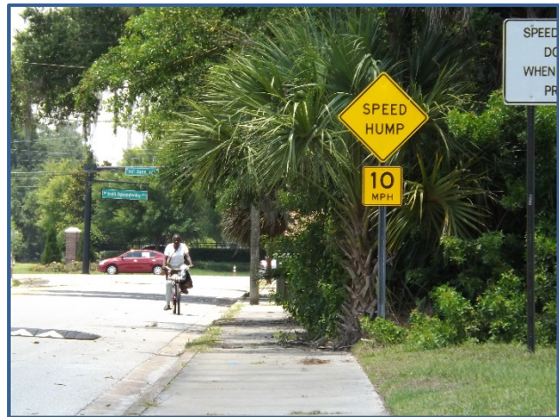
Vegetation obstructs the sidewalk on Adams St.
