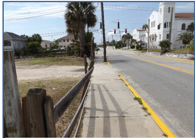
A damaged fence obstructs the sidewalk width on Grandview Ave.
