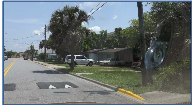
A gap in the sidewalk network along Walnut St.
