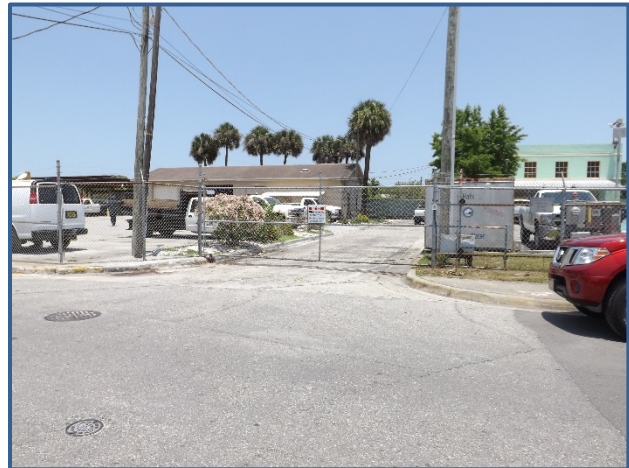
There are no ADA accessible sidewalk ramps in the 200 block of Marion St.
