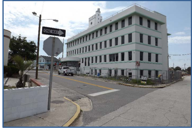
Sidewalk curbs lacking ADA accessible ramps at Coates St and Kemp Streets.
