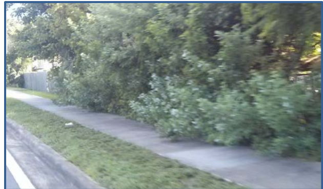
Vegetation reduces the useable width of sidewalks on SR 5A/Nova Rd.
