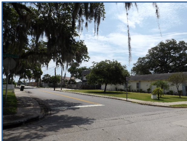
There are no ADA accessible sidewalk ramps at the intersection of Daytona St and Michigan Ave.
