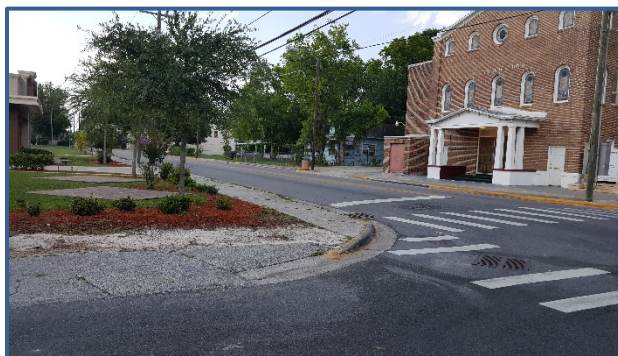
The west side of Loomis Street and Dr. MLK Boulevard lacks ADA accessible sidewalk ramps.
