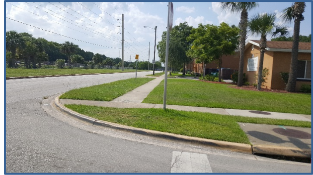
There are no ADA accessible sidewalk ramps at the intersection of Jean St and Loomis Ave.
