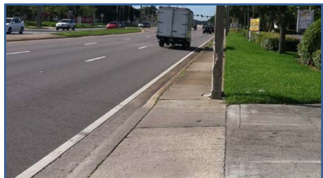
A utility pole located in the sidewalk at Midtown Plaza on SR 5A/Nova Rd.
