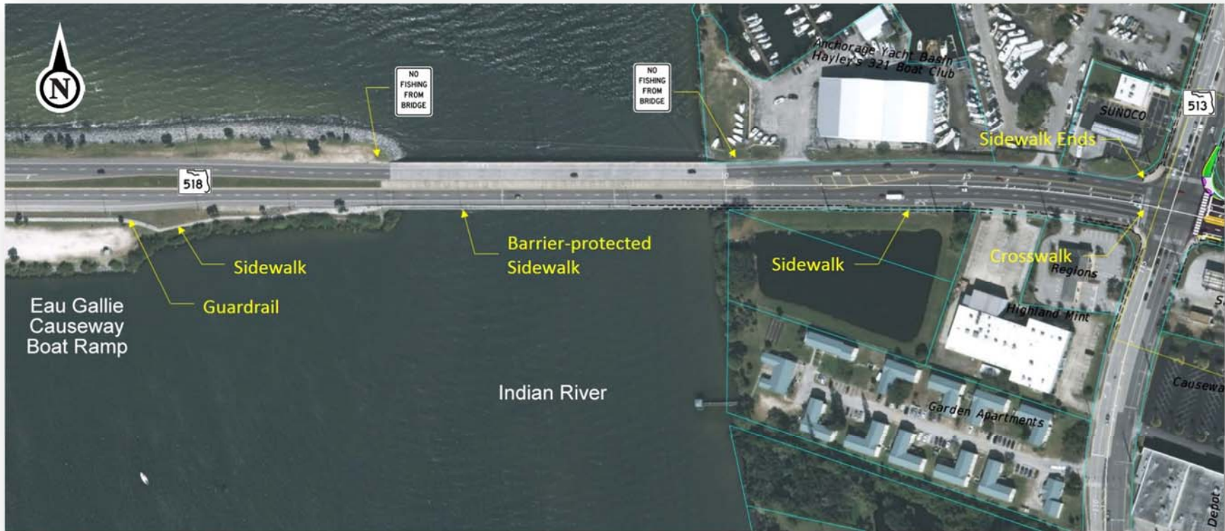
Figure 3.9 – Indian River Relief Bridge
