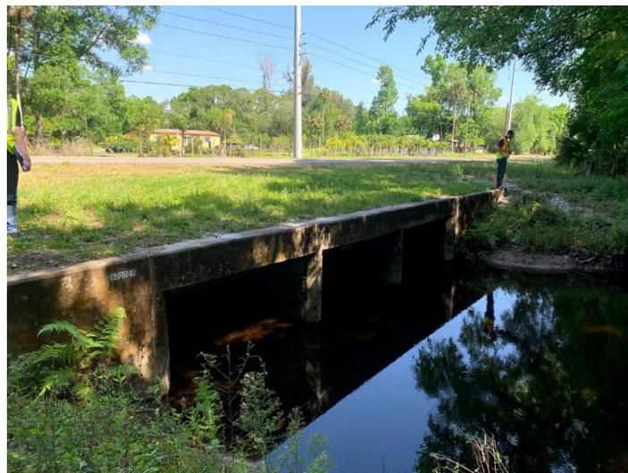
According to an above water bridge inspection dated 10/25/2019, the bridge is in good condition with a sufficiency rating of 90.8 and health index of 66.68. The existing load rating was performed via Load Test. The Minimum Inventory Rating Factor calculated is 0.85. No load posting is required.
