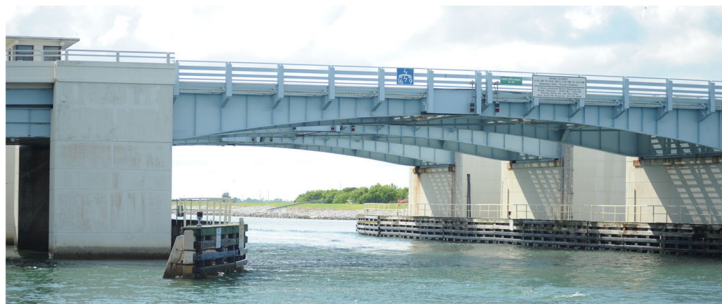
Figure 4-1: Existing S.R. 401 Bascule Bridges (No Build Alternative)
