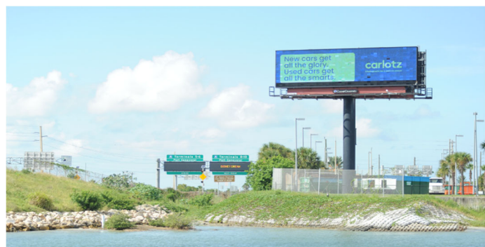
Figure 2-6: Existing Outdoor Advertising Structure
